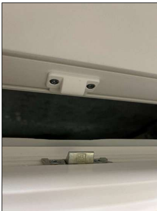
Photo 1: Restrictors in top frame and sash (DTI, 2022)
